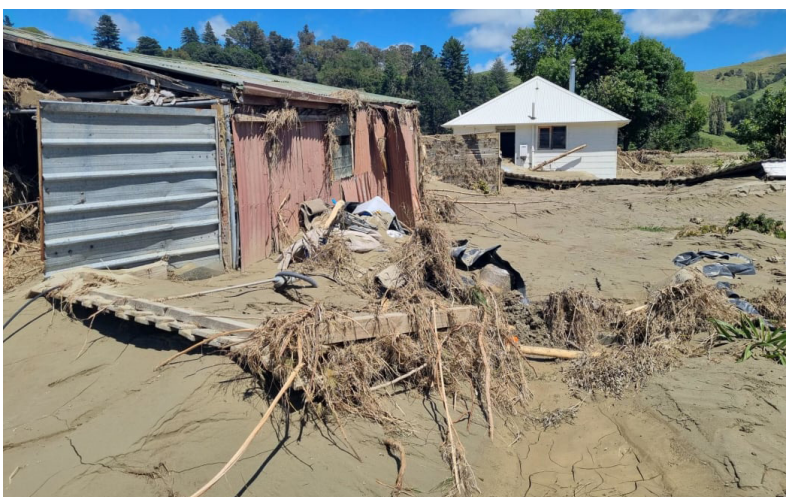
A property in Esk Valley after flooding caused by Cyclone Gabrielle, taken on Saturday 18 February. Photo: RNZ / Tess Brunton
